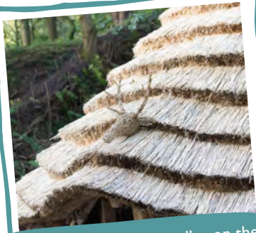
The layered thatch bundles on the roof of the Beeston roundhouse.
